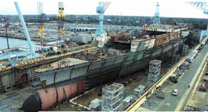
The aircraft carrier USS Ronald Reagan under construction, March 2000. (U.S. Navy)
